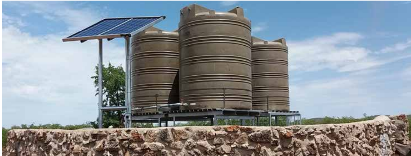
Fully equipped borehole with elephant wall
