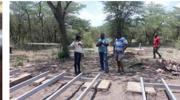
Onsite inspection: National and regional inspectors discussing the progress on site
