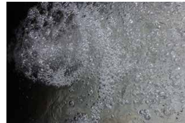
Water in a trough fixed to a concrete apron
