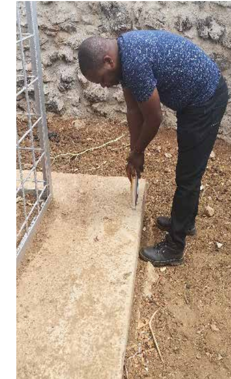
Testing concrete strength – 20mpa
