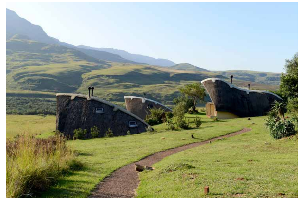
Didima chalets connected with footpaths leading to main reception
